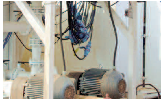
Electrical motors that operate on 440 VAC are among the equipment connected with the Deconnectors, which can be seen above.
