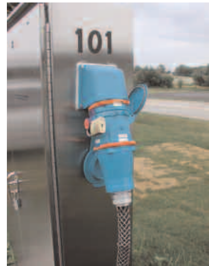
Unlike pin and sleeve devices, the Decontactor can be padlocked easily in the on or off position to eliminate the dangers of tampering.
