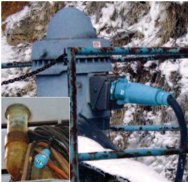
Float pumps or dewatering pumps can be safely and quickly disconnected and reconnected with Decontactors.
