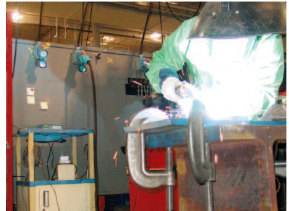
Three switch-rated welder receptacles provide power for Gas Metal Arc Welding in a EWI work cell.
