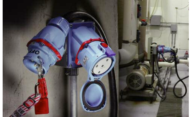
Decontactor plugs & receptacles can be easily locked out and tagged out.
