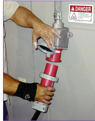
Most traditional plugs and receptacles should never be connected or disconnected under load.
